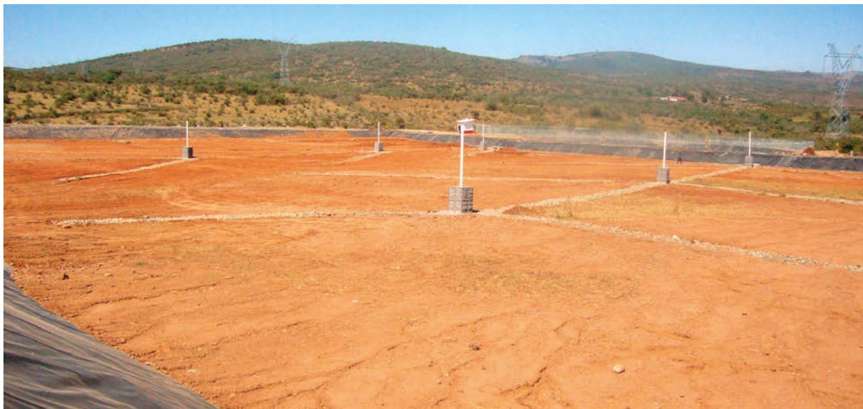
Relleno sanitario intermunicipal 2012
